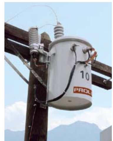
Single hanger bracket one high-voltage bushing self protected unit.
