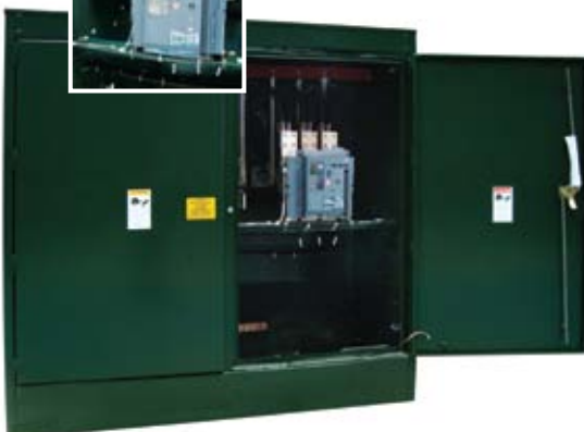
Low Voltage Molded circuit breaker installed in a plexiglass barrier
