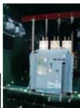
Low Voltage Molded circuit breaker installed in a plexiglass barrier
